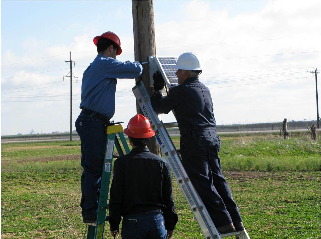
**Figure 8.3:** Workers installing the sensors on power poles at the Farnsworth, TX site. The nodes, equipped with special mounting brackets, were strapped to the poles with steel strapping. At the request of the site maintainers, great care was taken to not damage the poles.
